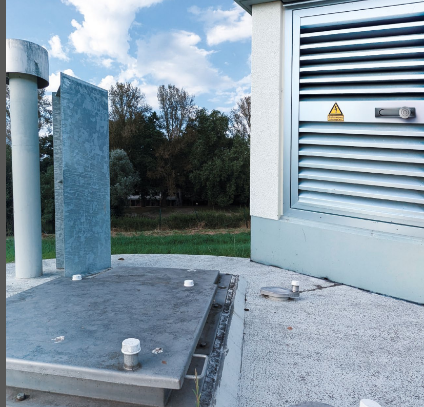
Manhole cover, type SD 7 load bearing
